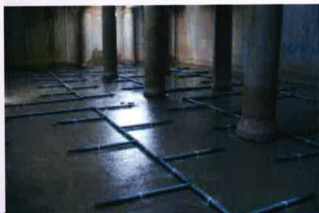
Underground Tank on piers completed
